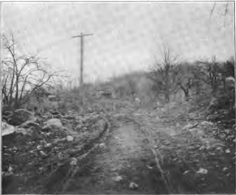
Stanhope and Newton road, Sussex Co., before improvement.
